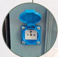
Electric control unit with 240V socket
